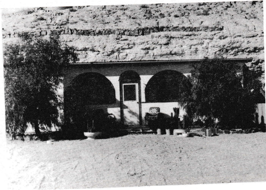
DUGOUT ENTRANCE WITH STONE BUILT UP ON FACE FRONT
