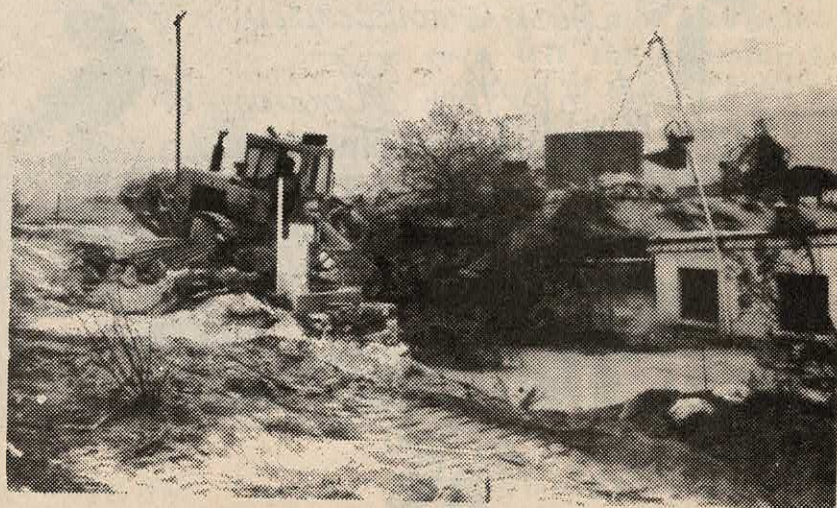
Demolition underway on the site
