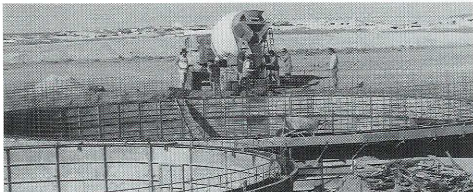
Contractors pouring concrete for the sewerage treatment plant
