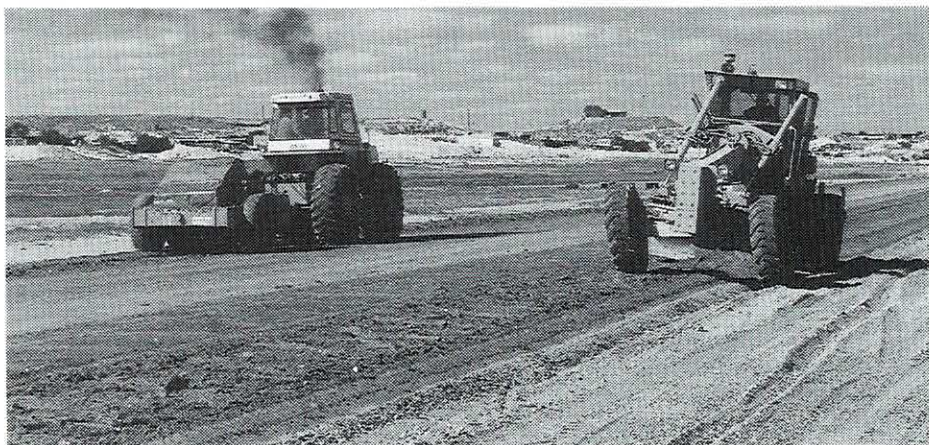
Earthworks on 17 Mile Road
