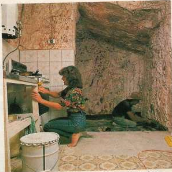
Rock-solid foundations and potential for modernisation: plenty of scope here for the DIY enthusiast
