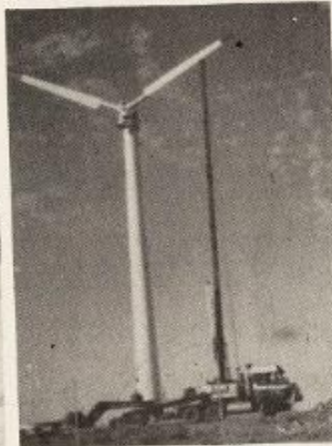
Hoisting the third blade into position
