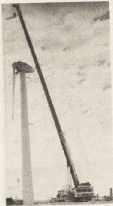
Installing the first 27 metre fixed pitch blade
