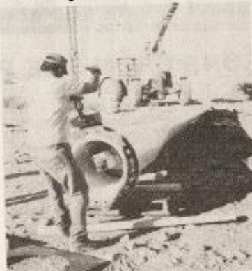
Harnessing the third blade for installation
